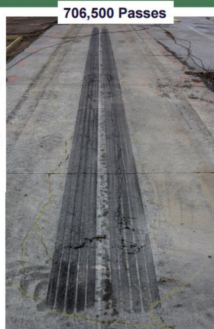
Pavement Condition at the end of testing
