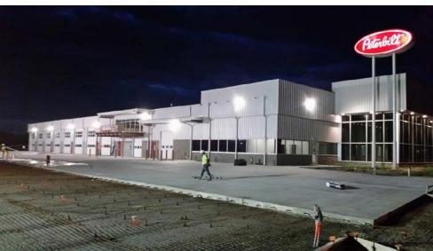
After considering the benefits of concrete over asphalt, Arscott selected concrete as the material for paving at the site. The pavement design was 8" thick with 6 gauge 4" x 4" wire reinforcement. The site concrete covered over 100,000 s.f. totaling over 2,700 cubic yards of 4,000 psi concrete.
