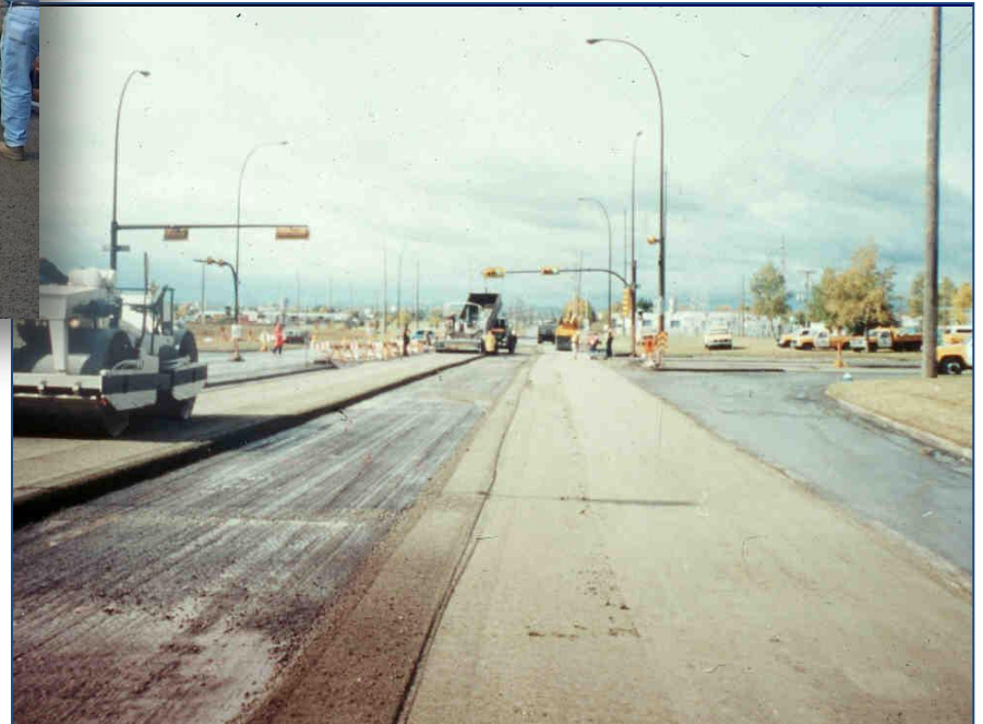
Intersection replacement Calgary, AB
