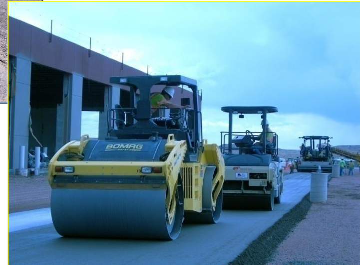
Fort Carson, CO 2008
