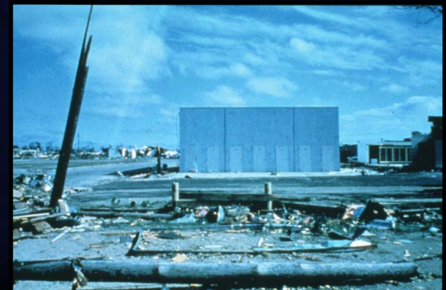
Walls standing after a tornado
