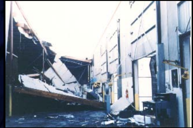
Walls standing after an earthquake
