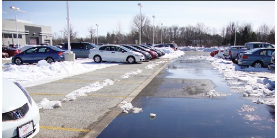
Pohanka Honda parking lot: pervious concrete on the left and asphalt on the right (see detail shot below-left).
