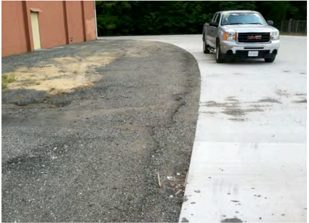
Above: Existing deteriorated asphalt paving side by side with new PCC. At right: Tammy Hill, Sales Manager at T&W Block in Onley, VA.
