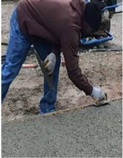
concrete should be placed with a semicircular motion with the chute. The less chute extensions the better to minimize drying out or getting held up coming out of the truck. Under the guidance of Bill Denison and Jim Murray, the contractors picked up the necessary skills to work with pervious concrete. This was a great example of the advisory council working together to promote technique in the industry for a shared customer.
