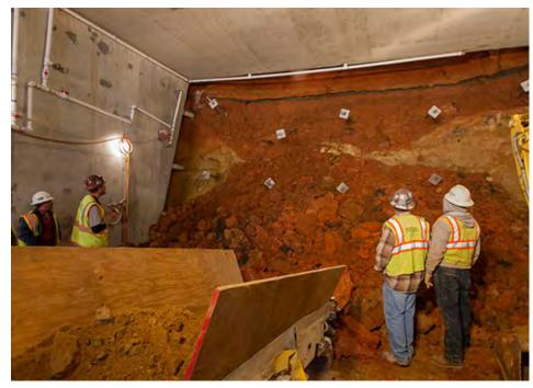
the earth immediately behind digging equipment so as not to weaken the support for trains passing overhead. Each tunnel box is pulled by six jacks and more than 160 cables, moving at one foot per hour when in full operation. The project will have used in the neighborhood of
