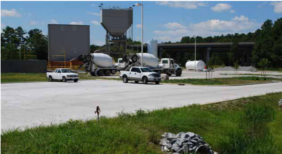
The Suffolk Ready Mixed Concrete is one of three certified Virginia plants.
