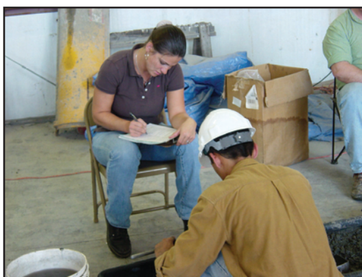
Angela Cable from VDOT Materials administers the slump test.
