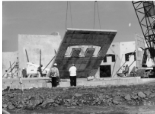
Tilt-Up Concrete workers construct a building in Northern Virginia.
