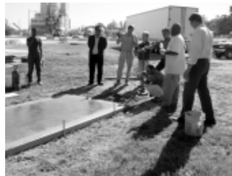
The finalization of the sidewalk is beginning to come into sight.
