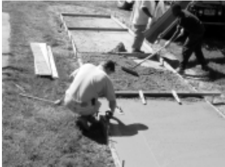
Contractors demonstrate the earlier stages of the process.
