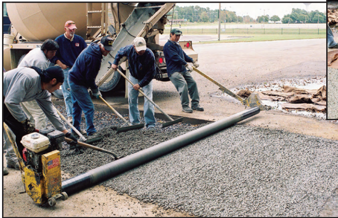
Placing the concrete.
