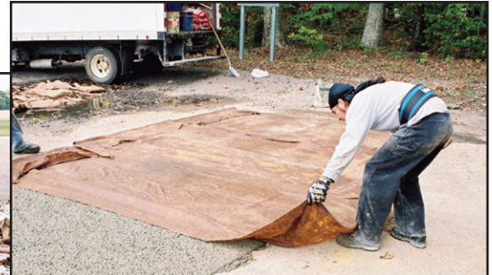
Curing the concrete.
