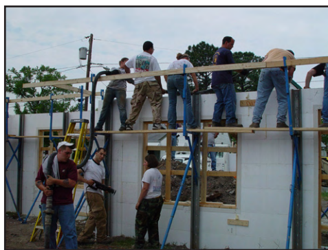
Workers at the site.
