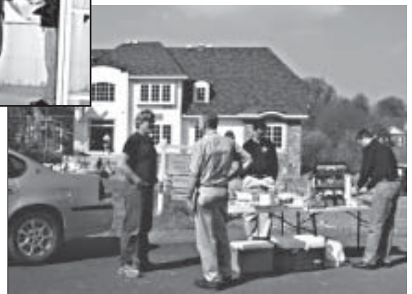
Top, the Angolia residence under construction. Bottom, builder J. P. Brehony talks with a client while Mike Renzi and Mike Newman set up the open house refreshments. Left, J. P. Brehony talks with architects about ICF construction techniques.
