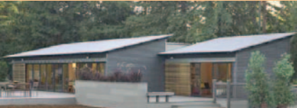
Exterior views of the Glidehouse home.
