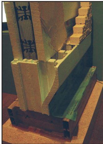
ICF Wall Panel Display in the Green House Building Exhibit at the National Building Museum.
