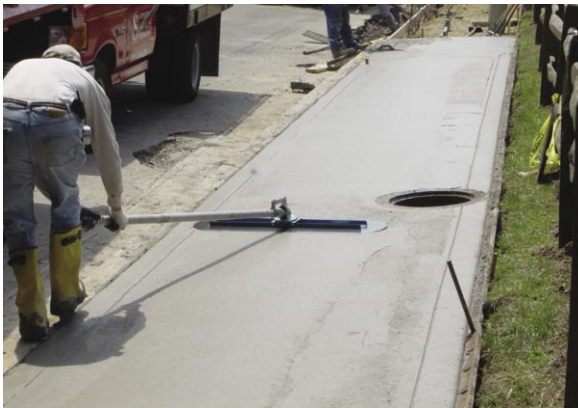
The construction phase of the project.
