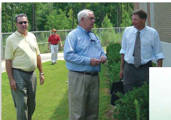
Inspecting the exterior walls.
