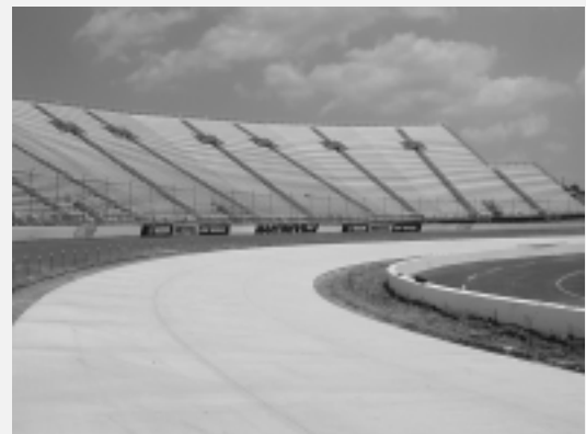
Completed concrete corner and turn at Martinsville Speedway.
