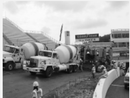
VRMCA member Boxley Materials delivers concrete for the repaving project.
