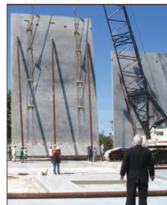
Reverend Falwell watches early panel erection.
