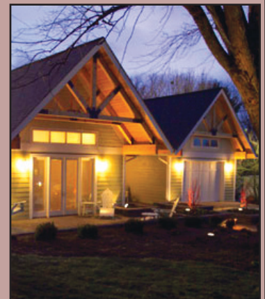
A nightly view of the completed Crawford-Smith home.
