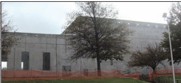
Church walls completed.
