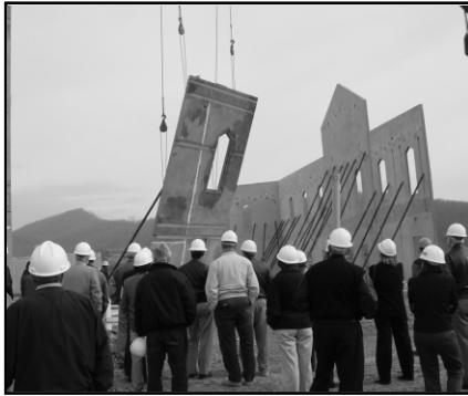
Attendees view the tilt-up construction demonstration.
