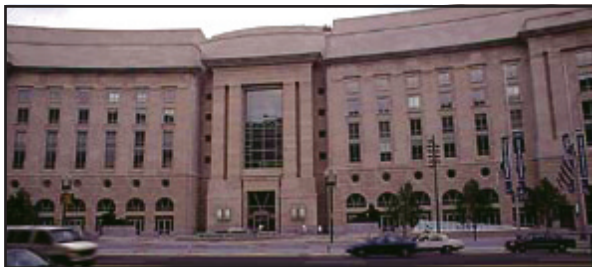
Reagan Building: View from 14th Street.
