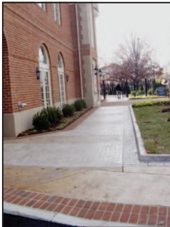
Walkway from the club house to the pool entrance.
