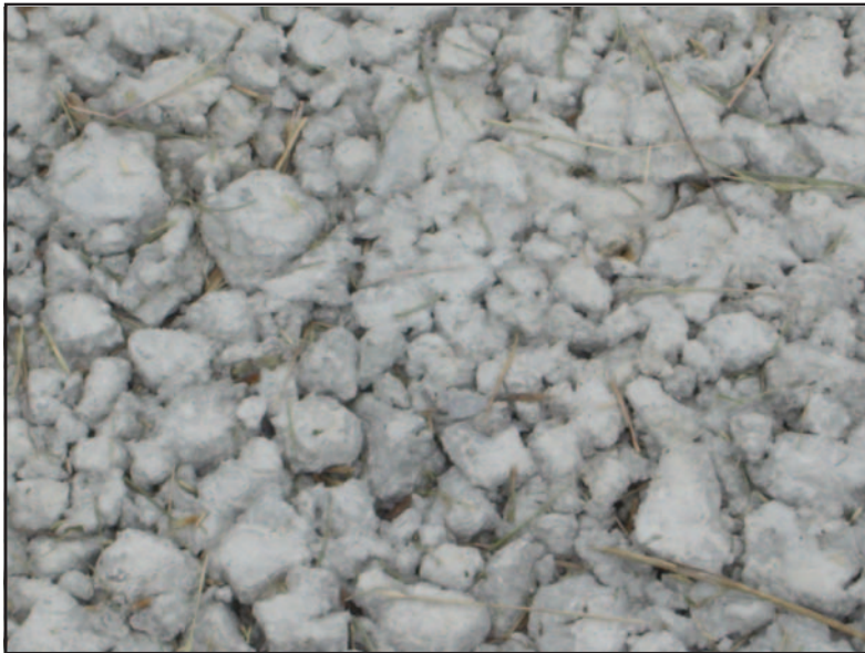
Close-up view of pervious concrete.
