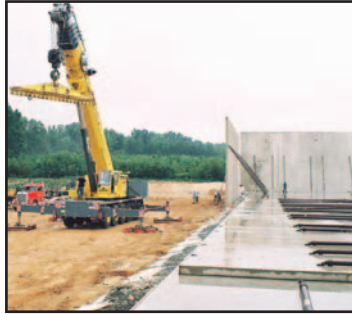
Crane in position to lift panels.
