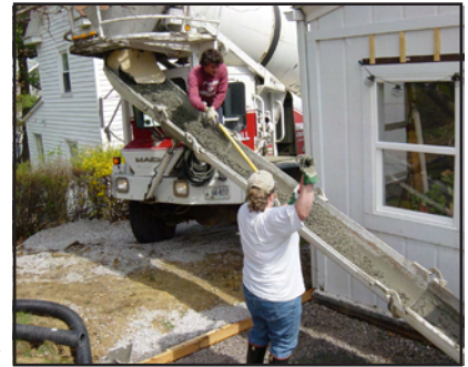
Mixer truck delivers to a difficult site.
