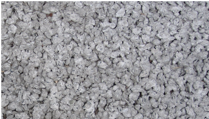
Pervious Concrete Parking at Food Lion Grocery Store
