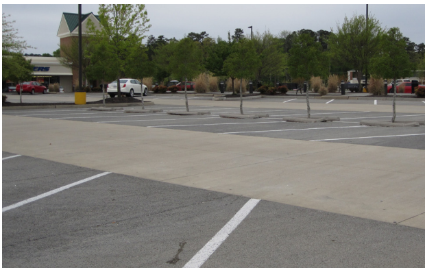
Pervious Concrete at Williamsburg Premium Outlets
