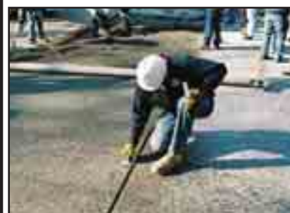
Finishing and edging the new panel with the previously poured sample.
